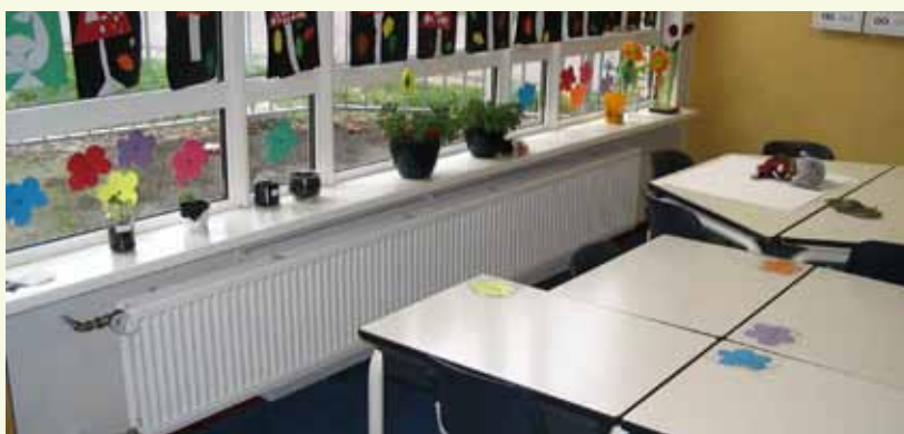
-Figuur 3- Climarad in schoollokaal (WTW)
